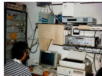
Control Room circa 1991
