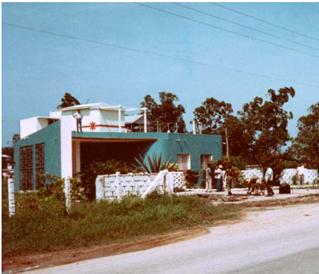
June 1977 SLR assembly (SLR housing, the white one with red star on door)
