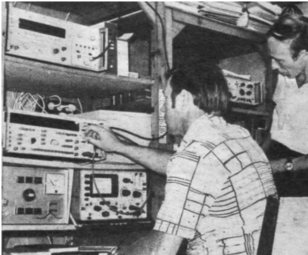
SLR control room circa 1890
