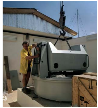
Assembly of the SBG system
