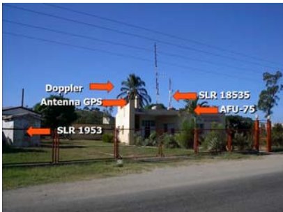
A view of the station with the systems locations
