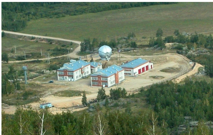
Figure 2. Current view of the Altay SLR station
