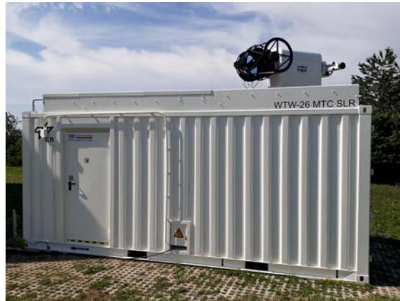
Fig. 1. STAR-C at the test site with raised platform.
