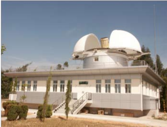
Figure 13-41. New Kunming SLR system facility.
