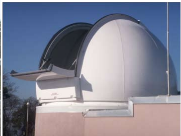
Figure 13-26. The new Graz SLR Observatory dome.
