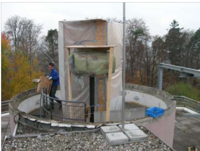
Figure 13-25. Dome replacement work.
